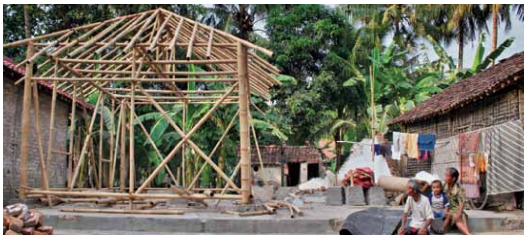
A transitional shelter built on the site of a destroyed house Photo: IFRC
